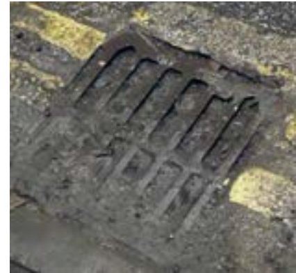
adequately maintain existing drains
